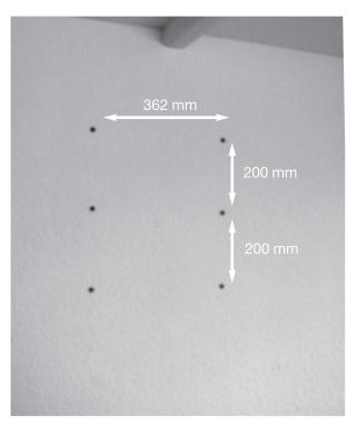
Decide where the wall mount is to be positioned and m ark the six fixture points. Take account of ceiling and head clearance. At least 10 cm (4") space must be left on both sides of the wall bracket to enable filter change within the bracket.
