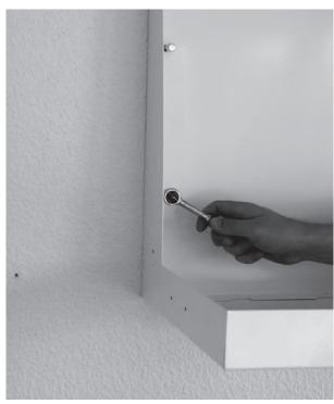
Tighten the screws with a 10 mm wrench. Do not exert vertical pressure on the bracket until all screws are securely in place.
